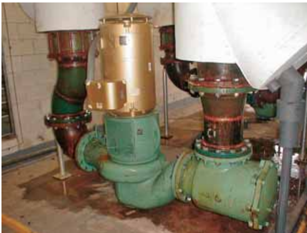
Chilled Water pump at Stephen P Clark
